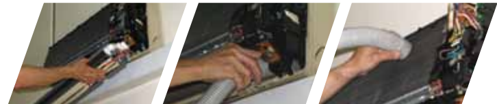
dismantle and clean water tray
